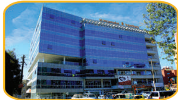
Arat kilo Building
